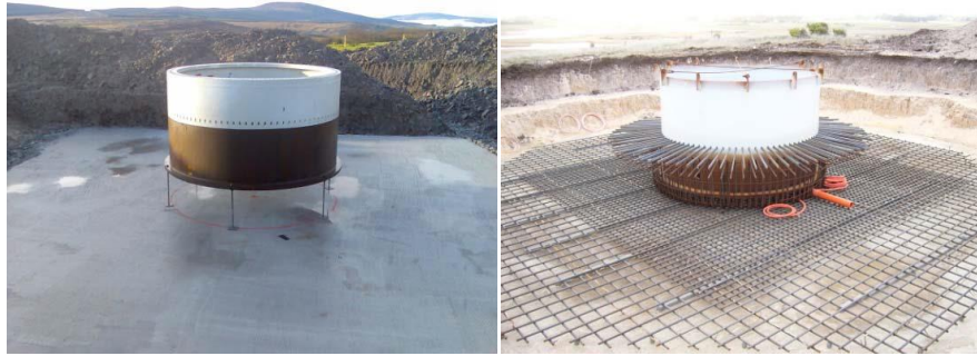
Plate 2.1: Levelled turbine tower “can”
