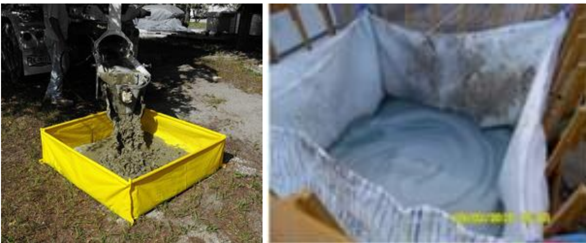
Photo 1 and 2 Example Photos of Concrete Washout On Site
