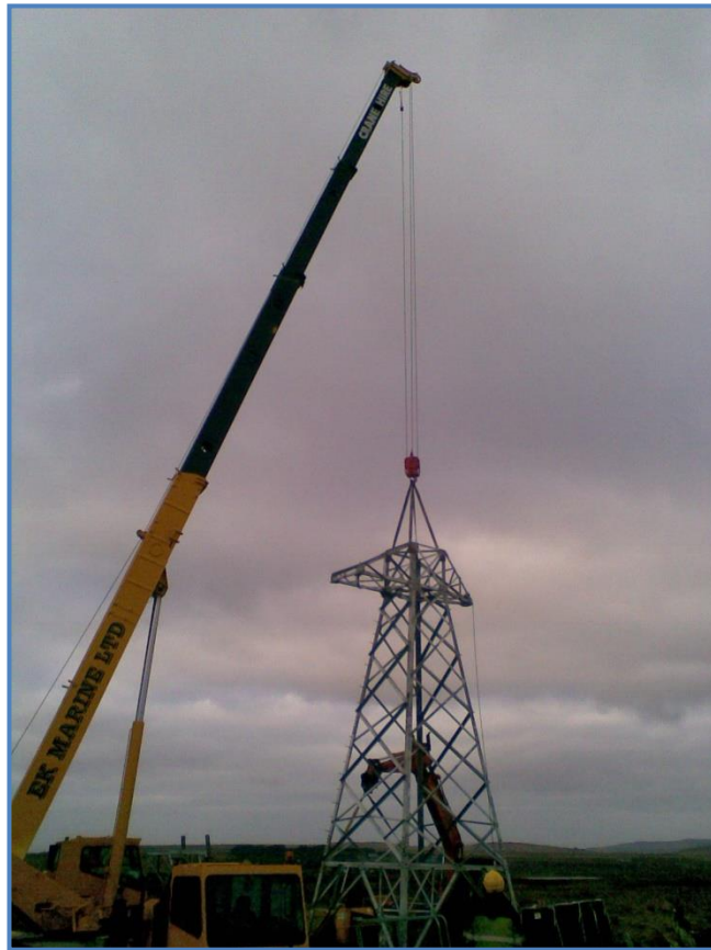
Plate 2.3: Angle Mast erection by mobile crane
