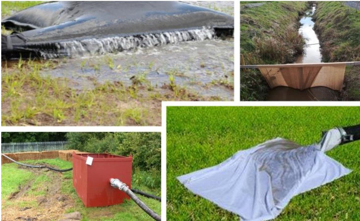
Figure 2.7: Examples of Proprietary Silt Control Measure
