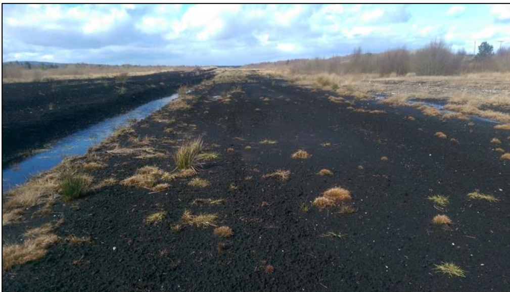
Plate 15.7: View of area of proposed internal haul road between turbines 1, 2 and 3, taken from the south.
